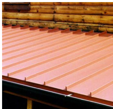
Standing Seam Mild Steel Roofing
