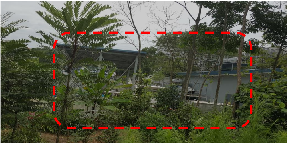
VIEWS /NOISE From Sub Station / Clean Energy Testbed
