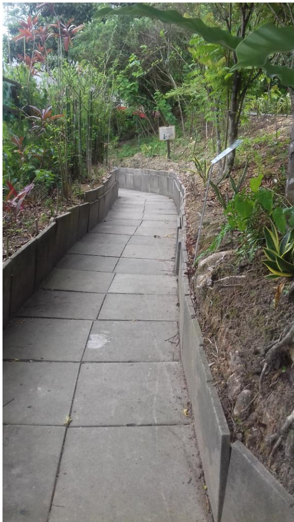
PEDESTRAIN CIRCULATION High use of concrete
