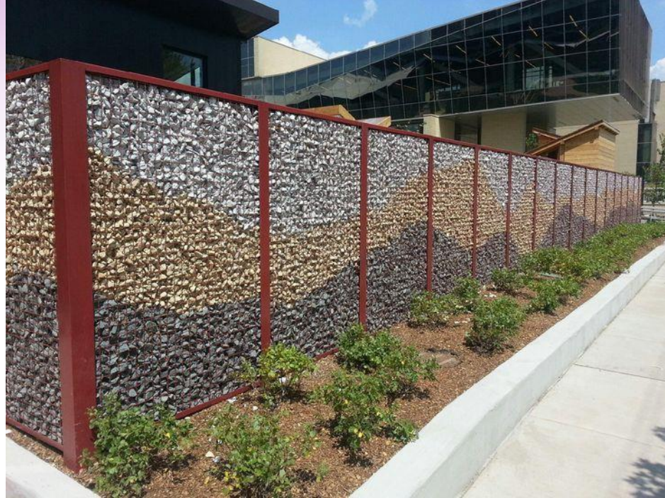
Gabion wall with layering of concrete aggregate of different colour
