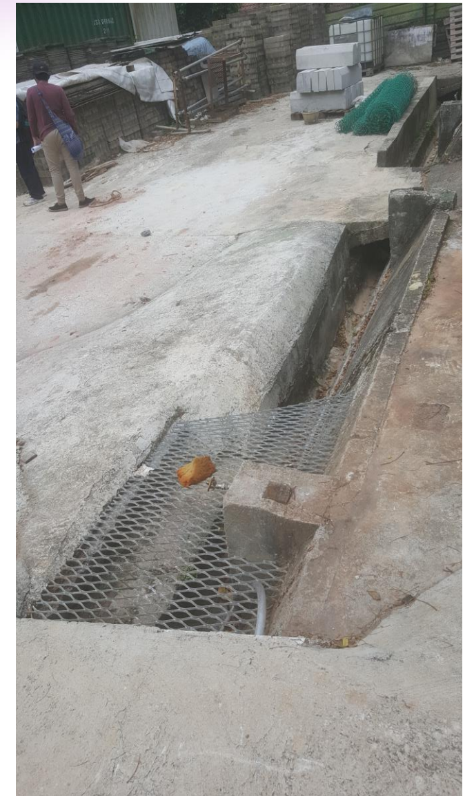
DRAINAGE Cover drains to remove falling threat
