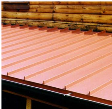
Standing Seam Mild Steel Roofing
